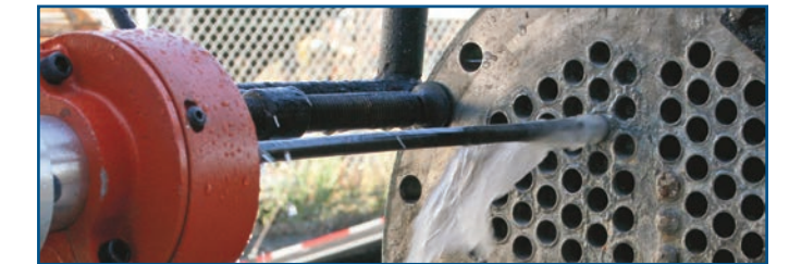
HydroDrill™ Tube Drilling
