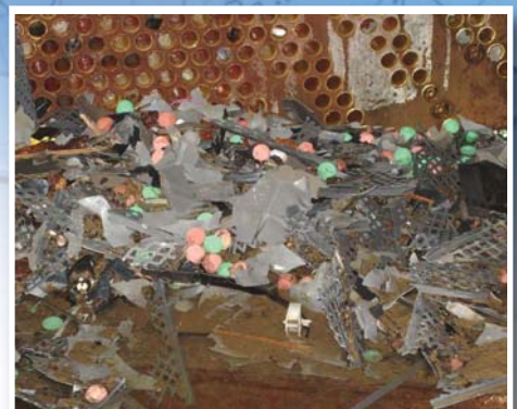
Some of the mud and debris removed from the water box condenser tubes using the Conco C45 tube cleaners.
