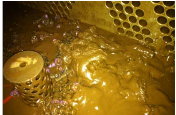
Figure 3. Mud and silt, particulate deposit as removed
