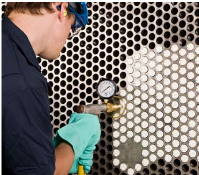
Figure 1. The heat exchanger cleaning process.
