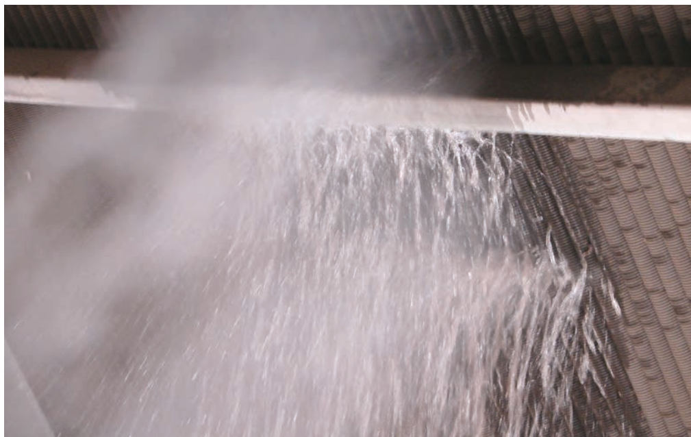
Back of Fins During Cleaning Operations
