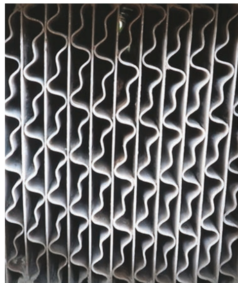
Preheater Basket After Cleaning with NitroLance
