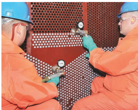
Conco Crew Shooting Tubes with TruFit Tube Cleaners
