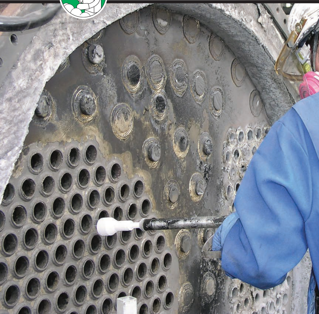
0.320" Thick Hardened Carbon Based Deposit
