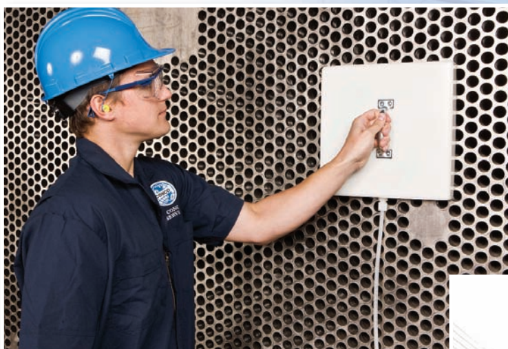
Conco technician conducts condenser tube leak inspection.
