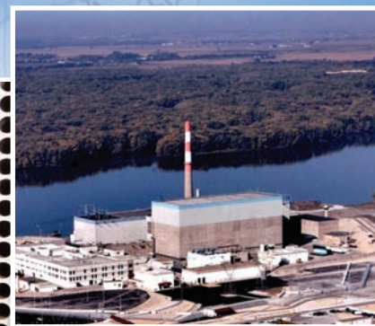
Quad Cities Generating Station, Cordova, Illinois.
