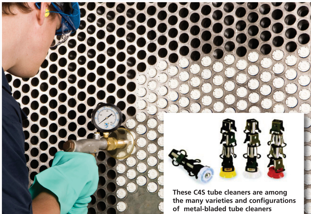
Conco technician "shooting" condenser tubes.
