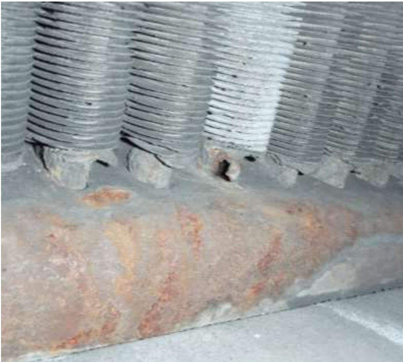
Holes in Tube Headers
