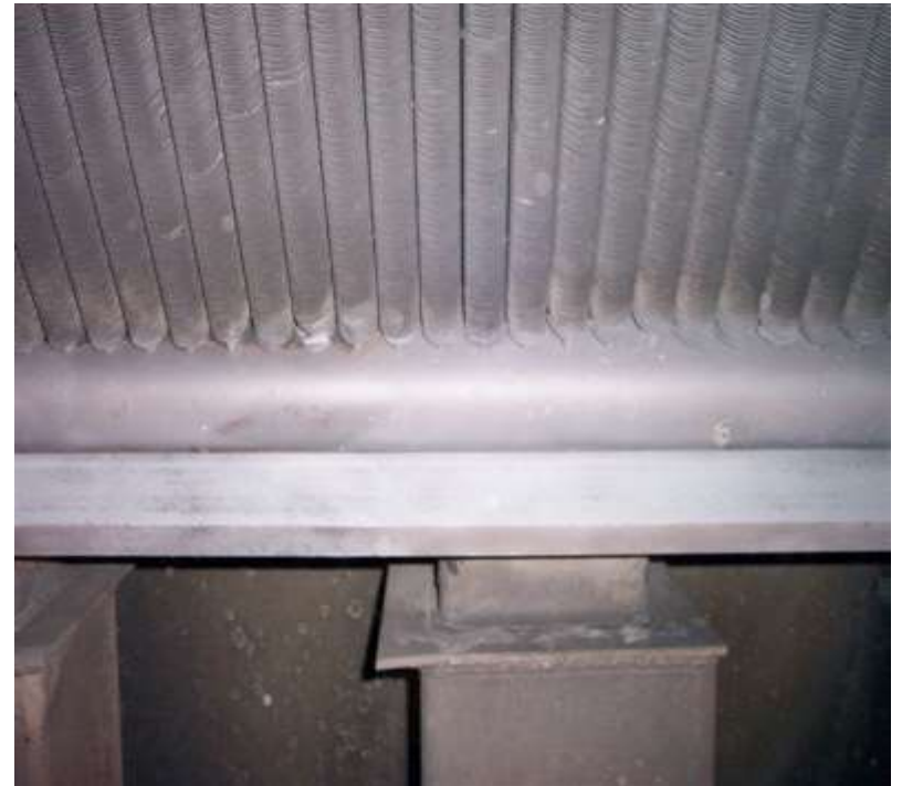
Holes Repaired and Epoxy Painted
