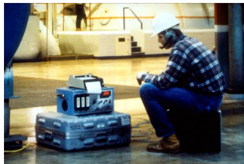
Figure 11 Technician at Monitor
